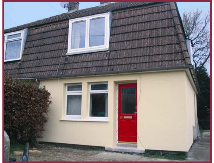
A refurbished 'Cornish' style home.
